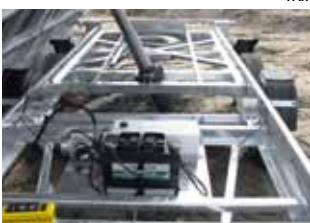
Electrical control of the hydraulic system
