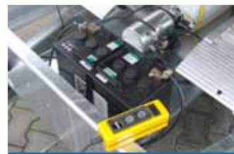
Electrical control of the hydraulic system
